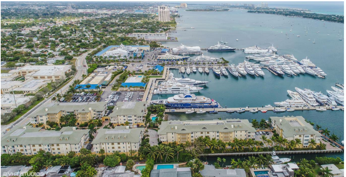
Figure 1. Aerial View of the Safe Harbor Rybovich Yacht Marina
